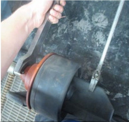
Fig 11. Install new main valve
