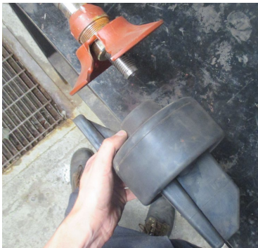
Fig 10. Remove main valve
