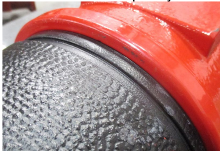
Fig 20. Ensure O-ring is covered at upper/lower barrel joint
